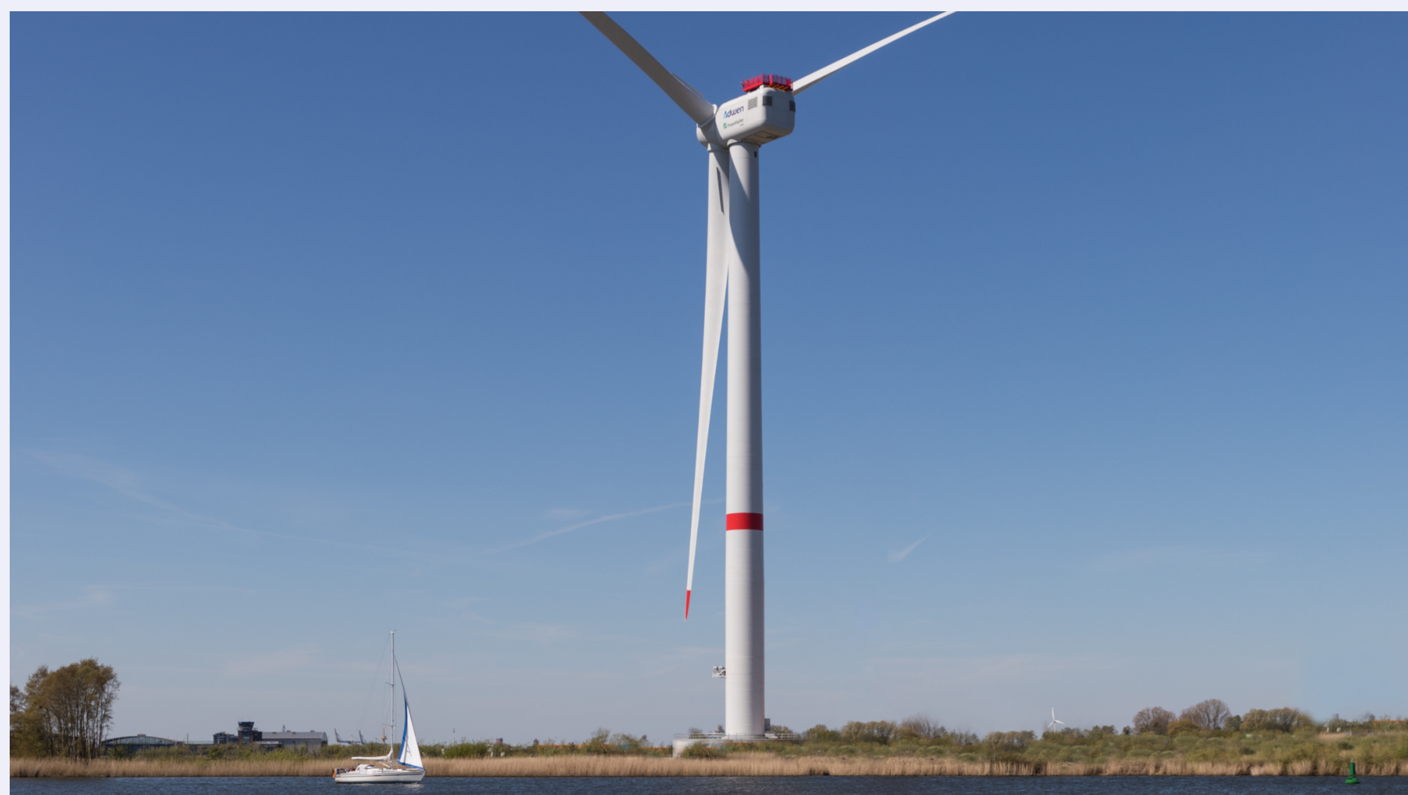
Prototype of the Adwen AD 8-180 wind turbine in Bremerhaven, Germany
